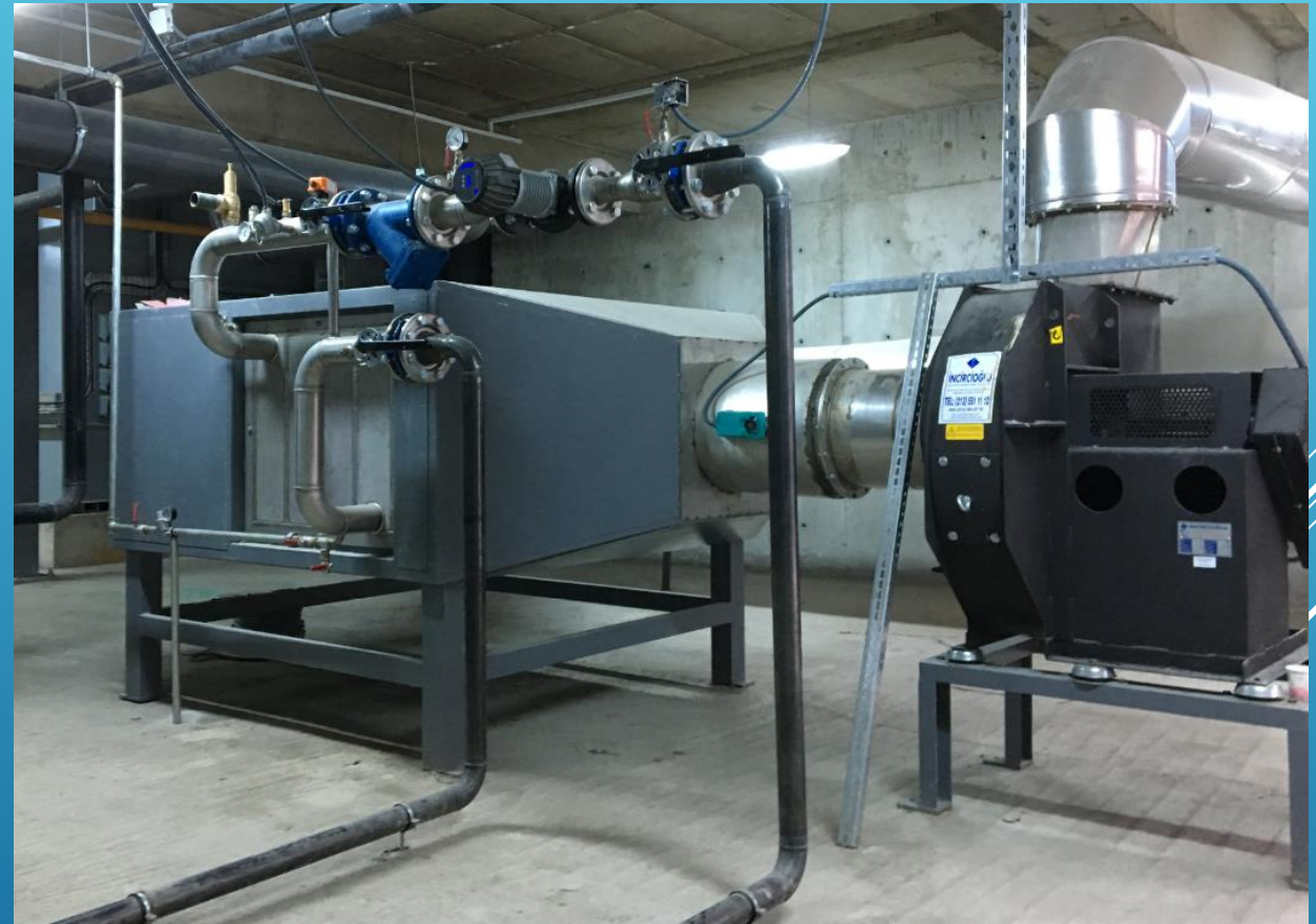
Heat Exchange System Air to Water
